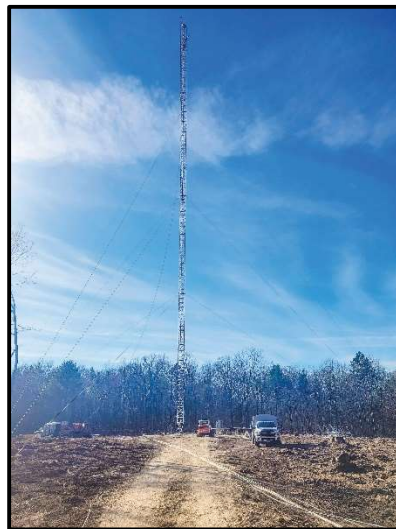
Figure 1: Cell Tower Installation
